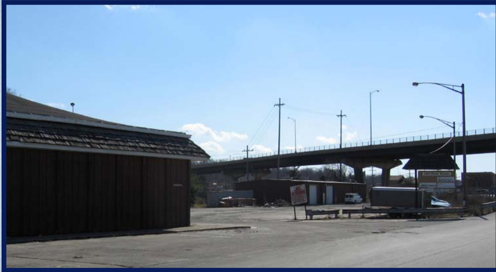
340 River Street “BEFORE”
