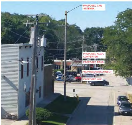
Figure 1 The previous 10 ft. height of the supporting equipment
