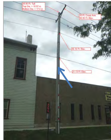
Figure 2 The blue arrow shows the approximate new 19 ft. location of the supporting equipment.
