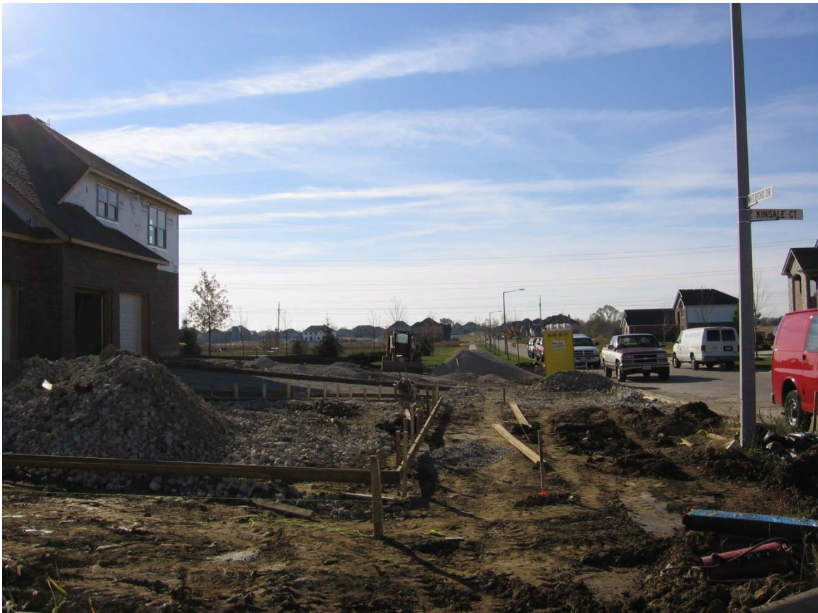
Subject Site – west side of lot
