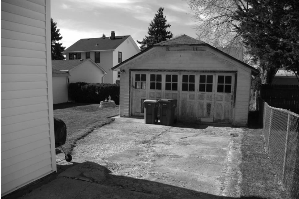
View of existing garage
