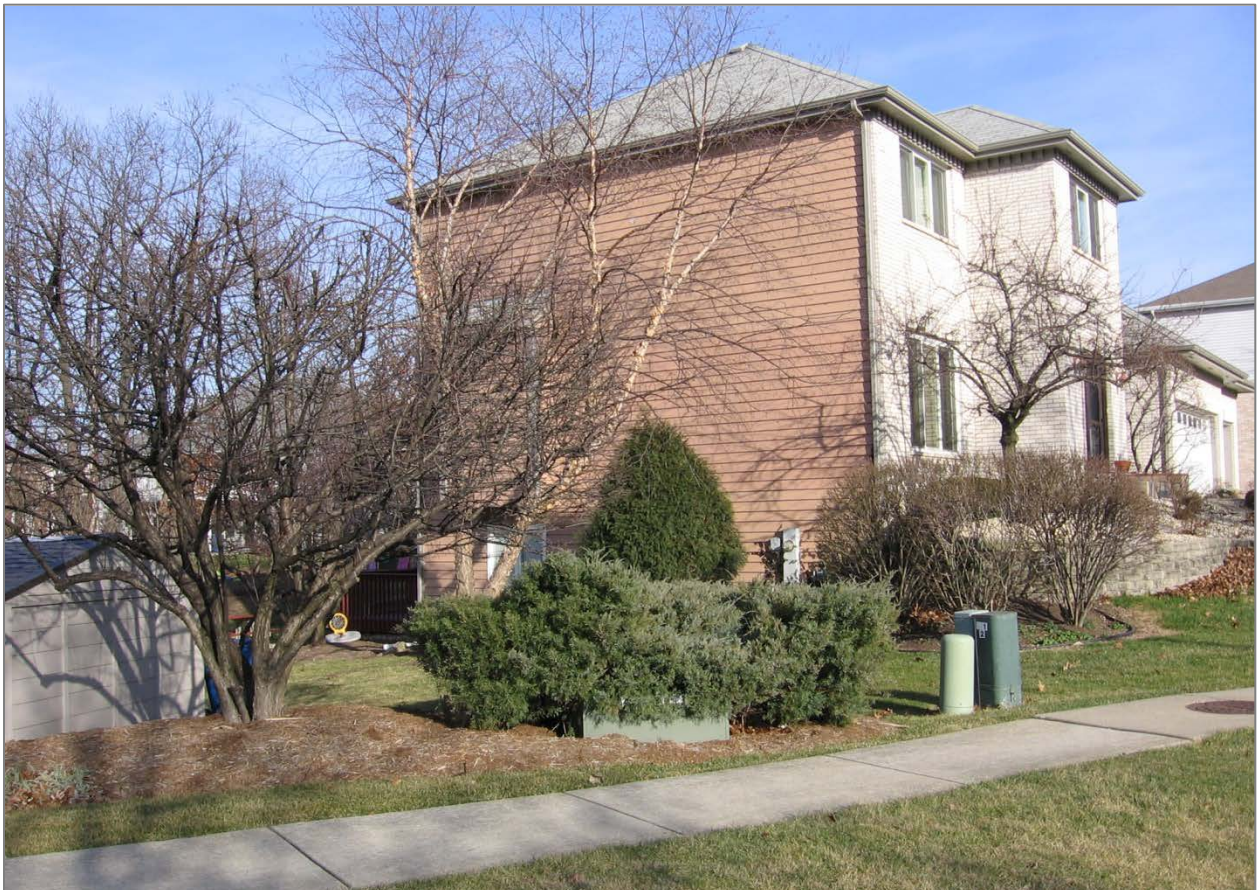
Shed and neighboring property to the east.
