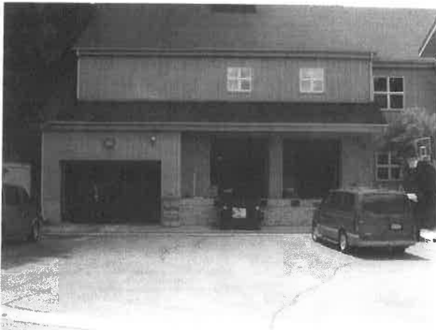
View looking west showing dock area along east elevation of cafeteria building
