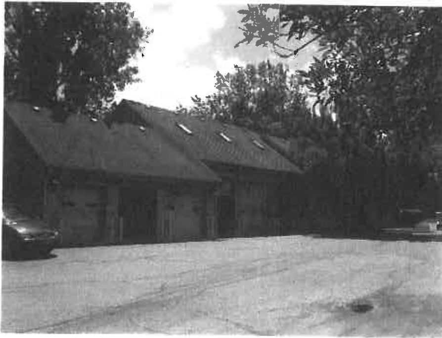
View looking southwest along north elevation of maintenance/garage facility (Building #11)
