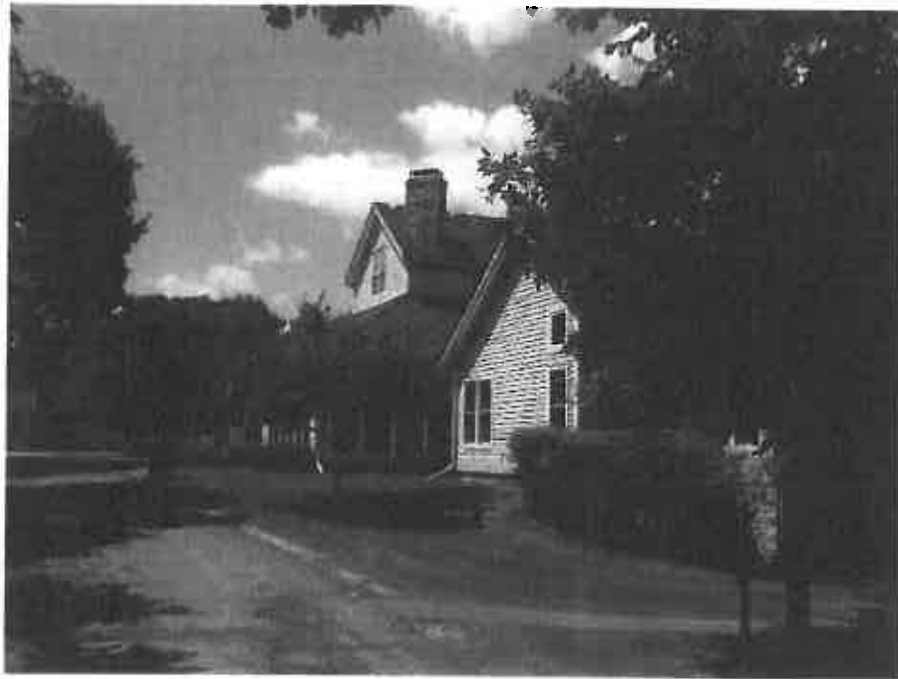
View looking northwest along south elevation of typical residential building (Building #5)
