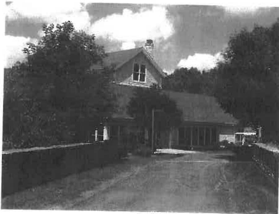
View looking northeast along south elevation of typical residential building (Building #2)
