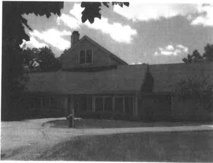
View looking west at east elevation of typical residential building (Building #3)
