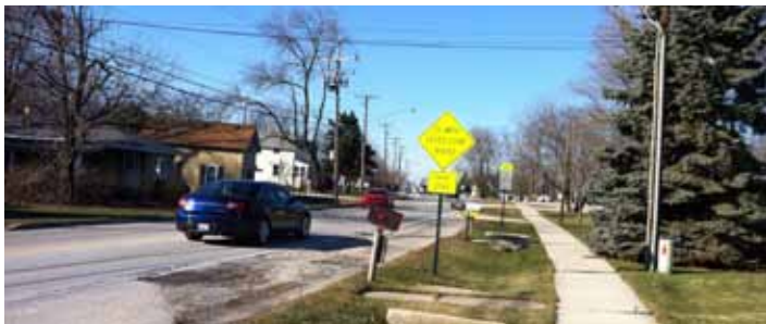
Crossing busy streets like McCarthy Road can be a barrier to walking or biking to school.
