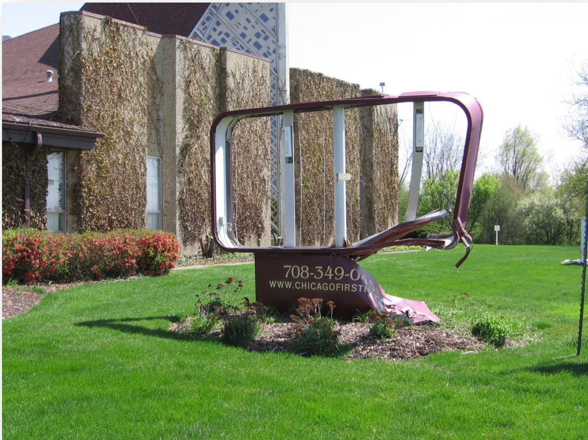
Existing, damaged sign
