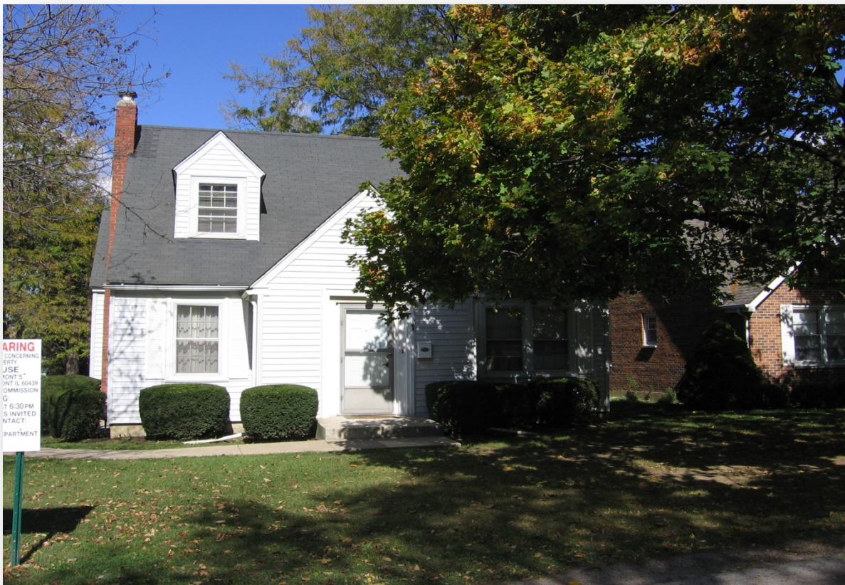
Subject Site, as viewed from Povalish Court
