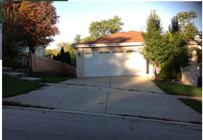
Figure 2 Home to the north of subject property
