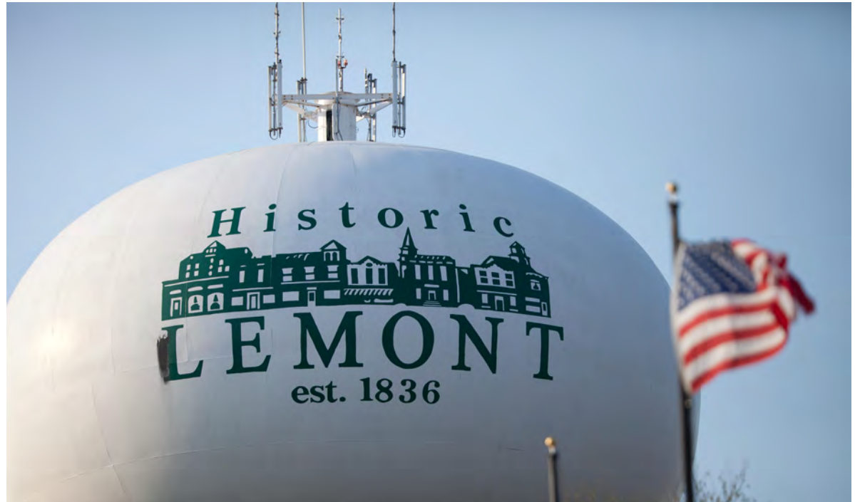
Lemont is one of the few communities in the area to rely on groundwater for its public water supply; many surrounding communities rely on Lake Michigan water.
