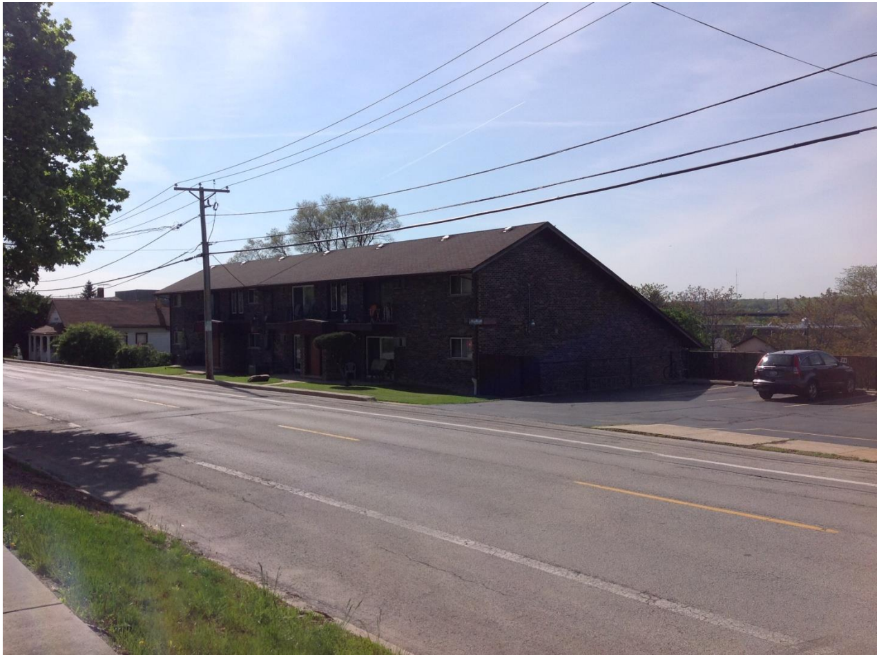
Figure 3 Multi-family structure along the north side of Illinois Street.
