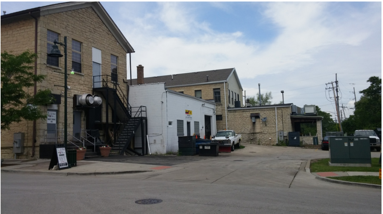
Figure 2 Rear façade and alley
