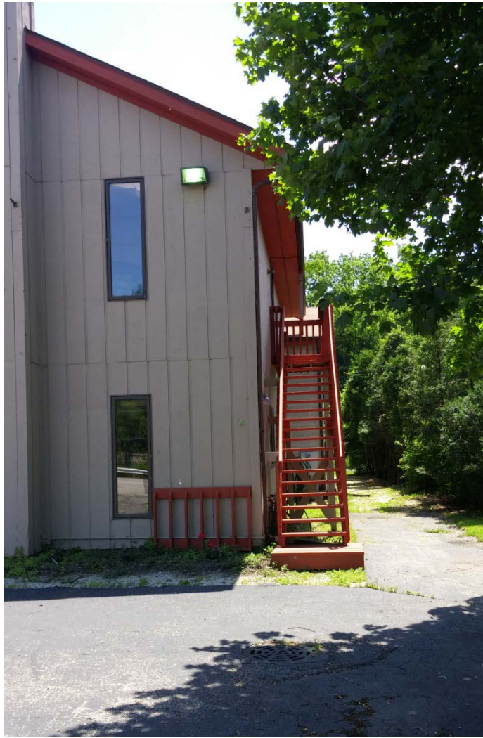
Figure 3 Second floor side entrance.
