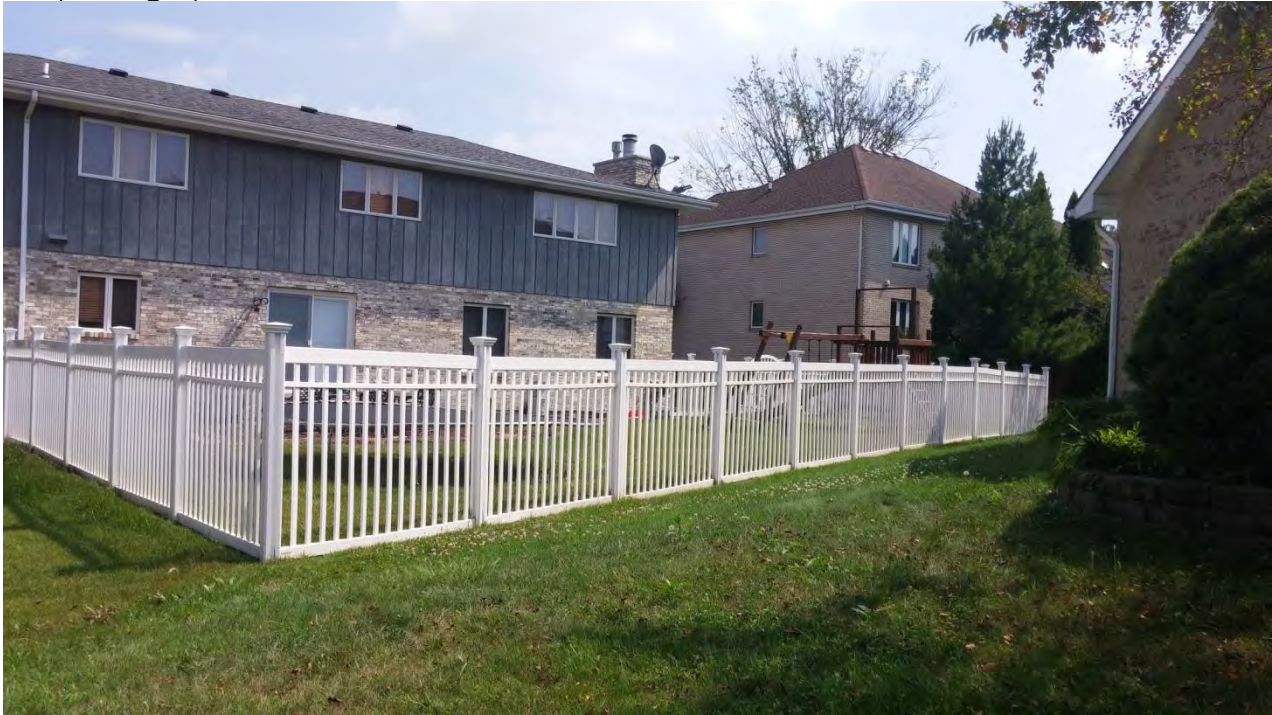
Figure 1 View from neighboring driveway
