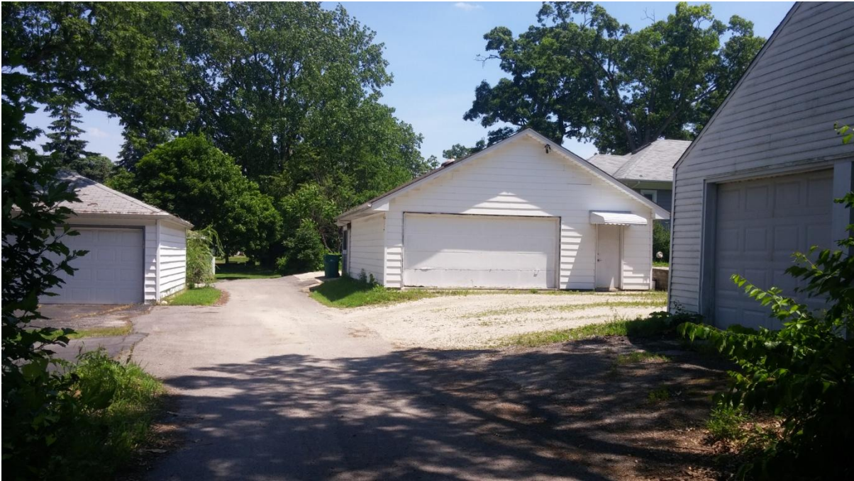
Figure 5 Neighboring properties to the west of the subject property whose driveways access from the alley.
