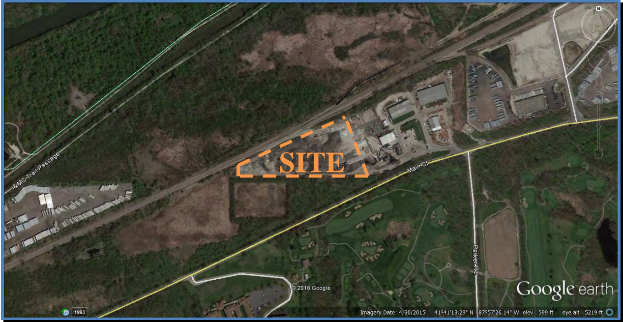
Aerial View of Proposed Facility
