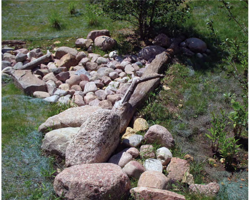
Figure 1-9: Rock check damn
