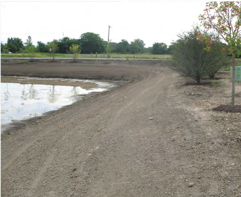
Figure 3-6: Acceptable prepared site
