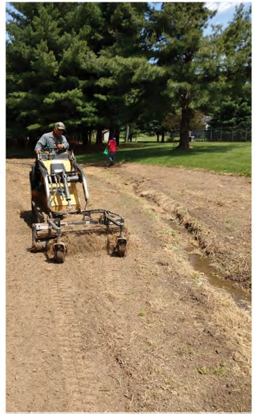
Figure 3-7: Removing debris & prepping site
