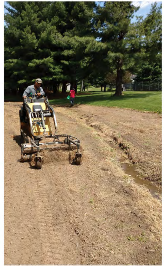
Figure 3-7: Removing debris & prepping site
