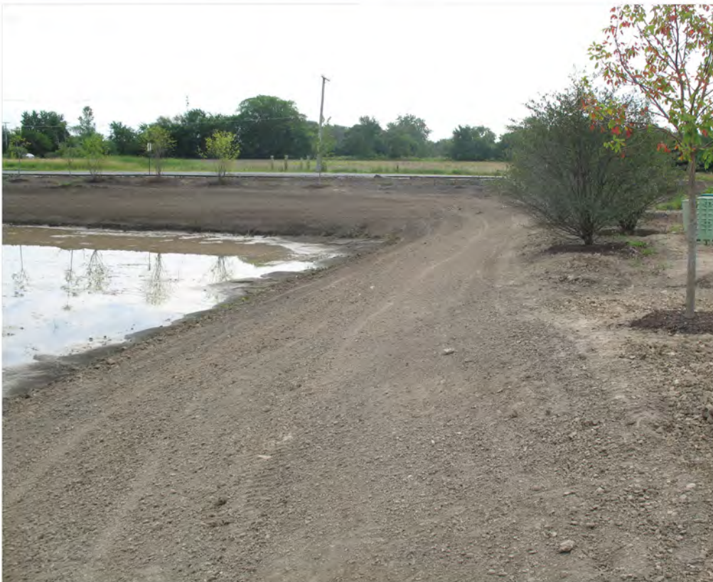
Figure 3-6: Acceptable prepared site
