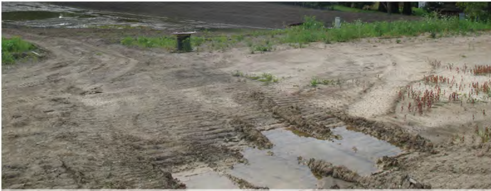
Figure 3-5: Ruts in the soil to be smoothed
