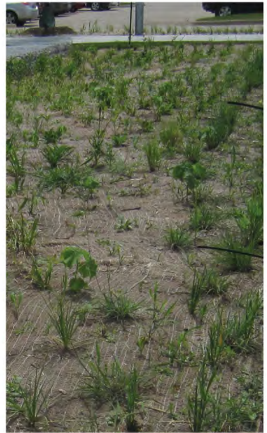
Figure 3-17: Plugs planted in erosion blanket
