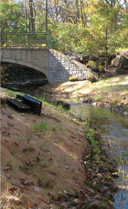
Figure 3-18: Erosion control blanket on a slope
