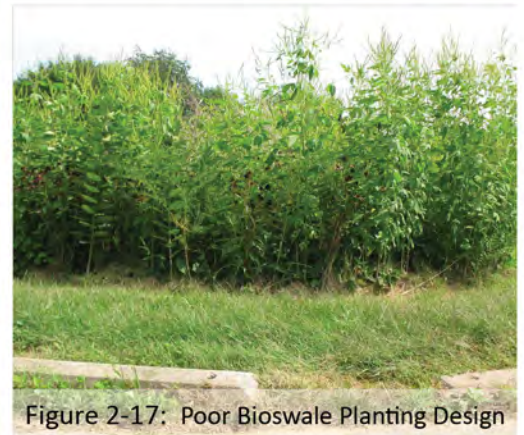
Figure 2-16: Poor Bioswale Planting Design
