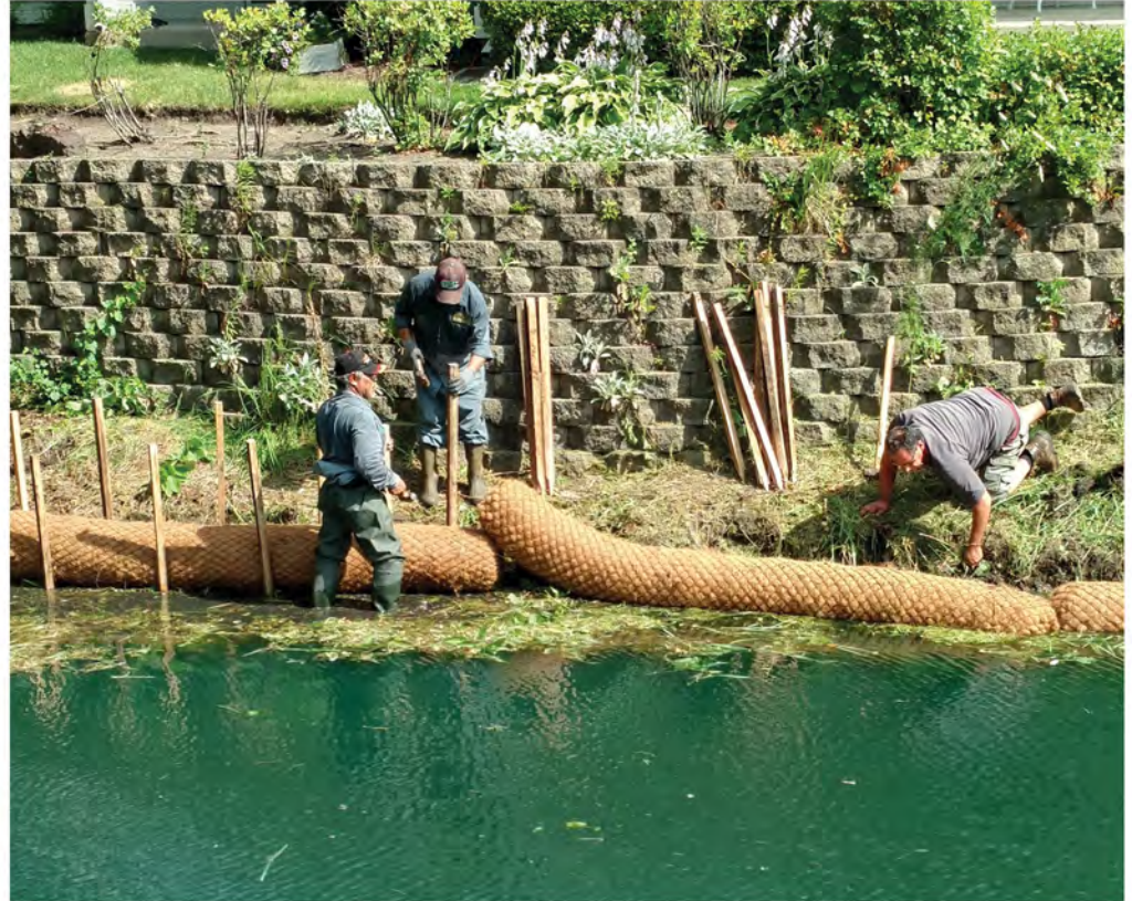
Figure 3-19: Coir log being installed along a stream bank to hold grade
