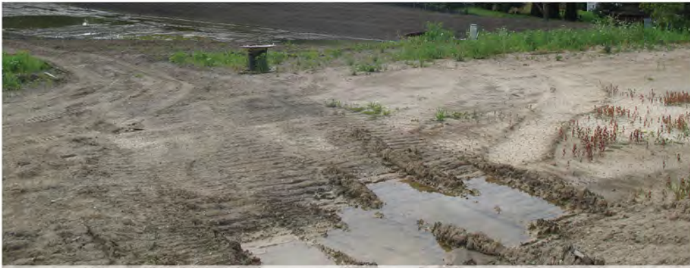
Figure 3-5: Ruts in the soil to be smoothed
