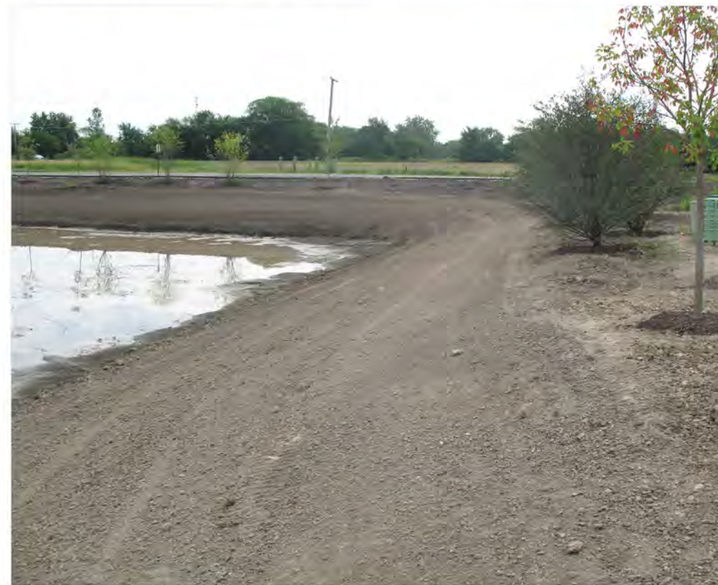
Figure 3-6: Acceptable prepared site
