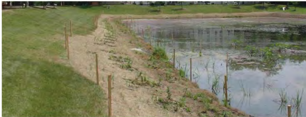
One week after planting - Photo illustrates goose exclosure, erosion control blanket, shoreline plug planting, and aquatic plug planting (July 2004).
