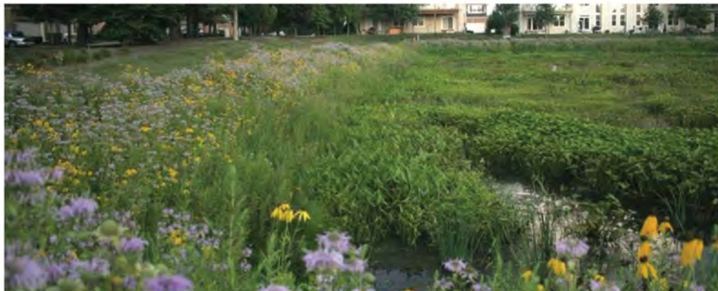
Two years after planting - There is a beautiful and functional wildflower and wetland planting that serves as habitat for local wildlife. The wetland plants cover the basin bottom and increase water quality (July 2006).
