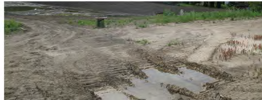
Figure 3-5: Ruts in the soil to be smoothed
