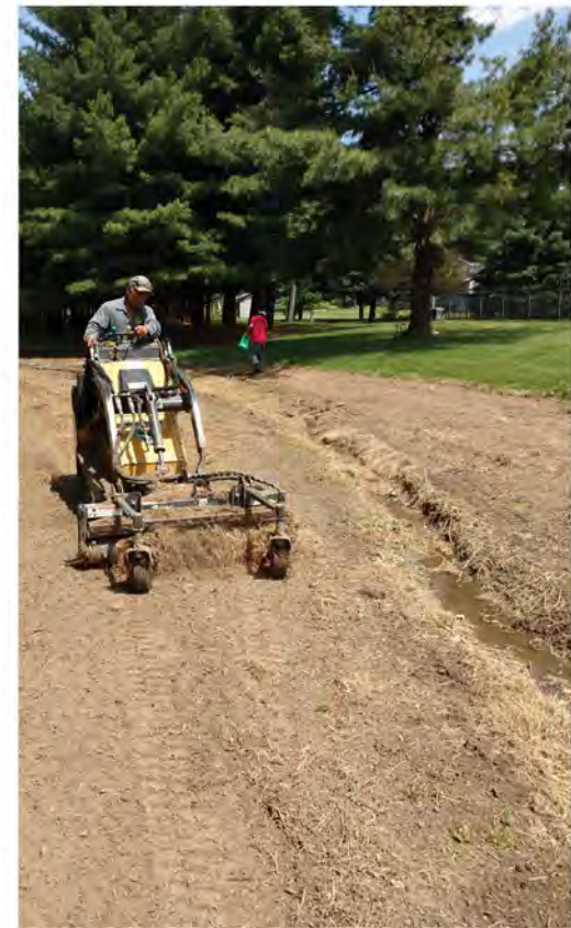
Figure 3-7: Removing debris & prepping site
