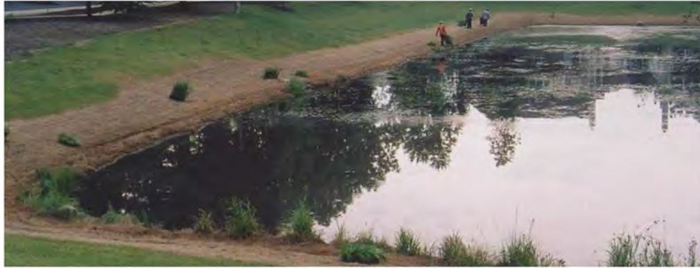
Existing Conditions - A retention basin "Green Retrofit". Planted in July 2004, notice there is nothing growing in the water.
