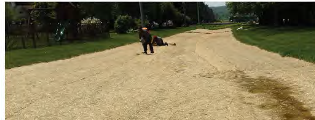
Figure 3-17: Hand seeding over a straw erosion control blanket
