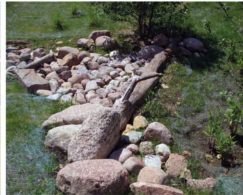
Figure 1-9: Rock check dam
