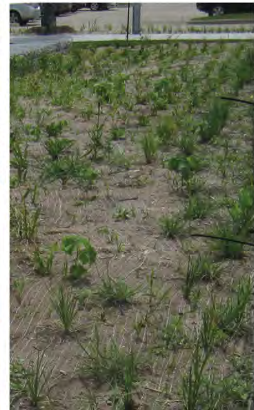
Figure 3-18: Plugs planted in erosion blanket
