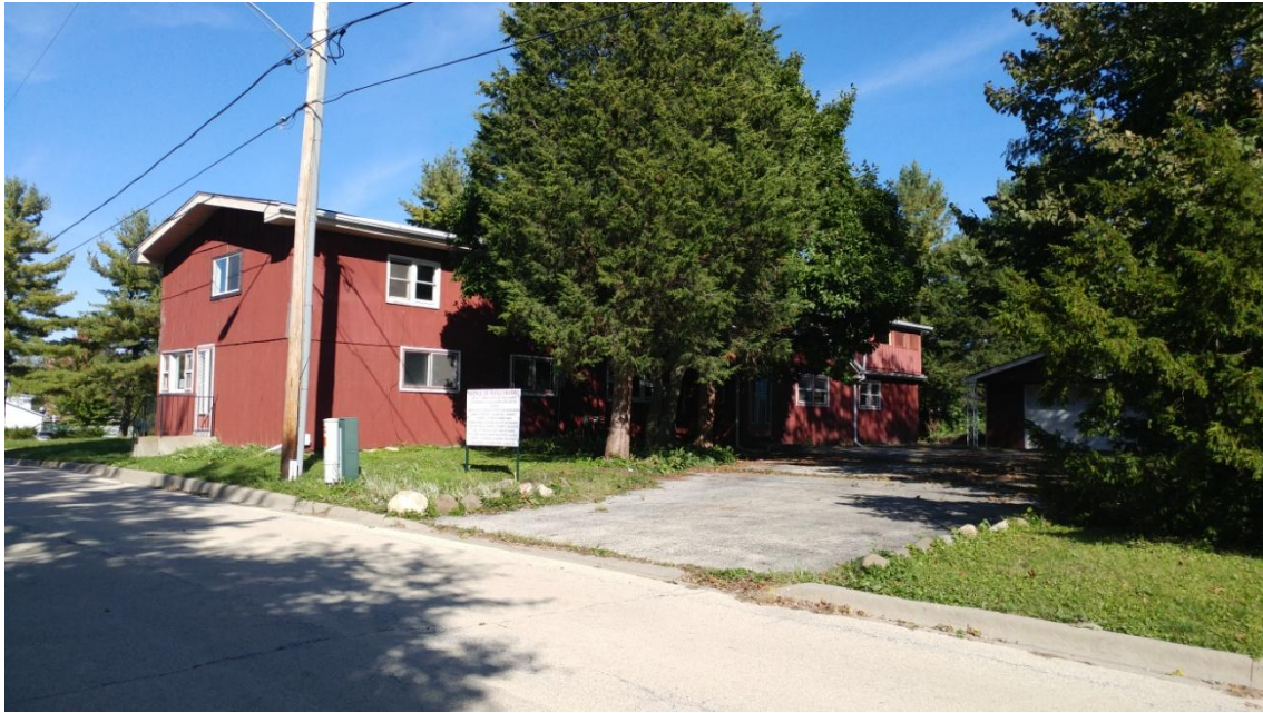
Figure 3 The existing home's entrance sits 9 ft from the street. The stairs to the front entrance sit only 5 ft from the street.
