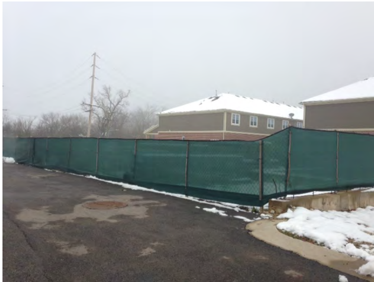
Figure 2 In 2006, the applicant poured the foundation for building C as an eight unit. This foundation is proposed to be converted to seven units.
