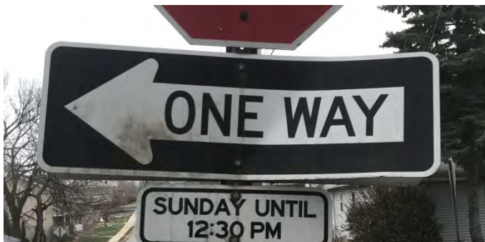
Figure 1 This is an example of the staff recommended sign for the proposed east entrance driveway. The left turn restriction can be limited to Sunday morning.
