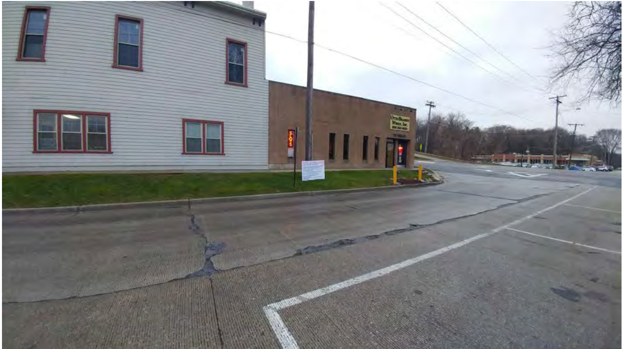
Figure 1 Pedestrian's view of the ComEd utility pole looking south.
