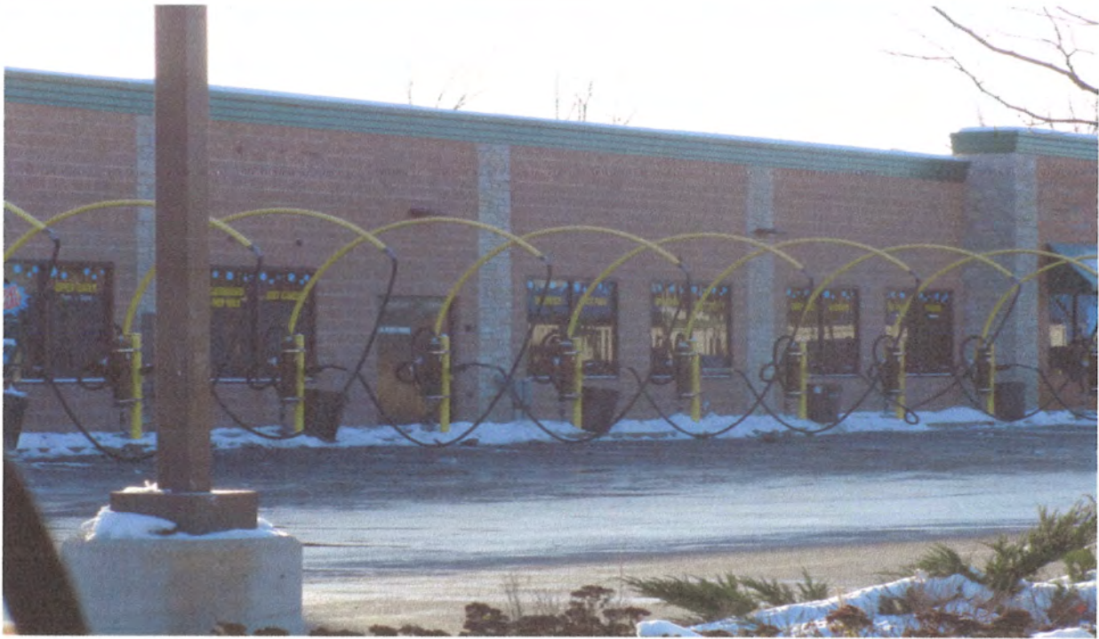
EXAMPLE OF VACUUM SYSTEM OF OTHER CAR WASH – STATE STREET VIEW
