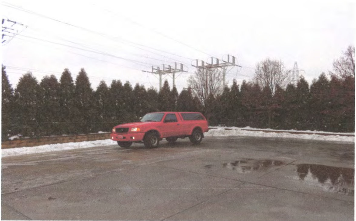
S. W. CORNER VIEW - CAN NOT SEE COMED SUB STATION, OFFICE MAX OR RESIDENCE DUE TO MATURE LANDSCAPE
