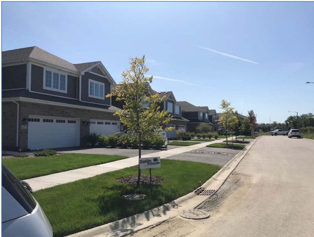
Figure 3: Looking down Lacey Drive at completed Buildings 2 and 4
