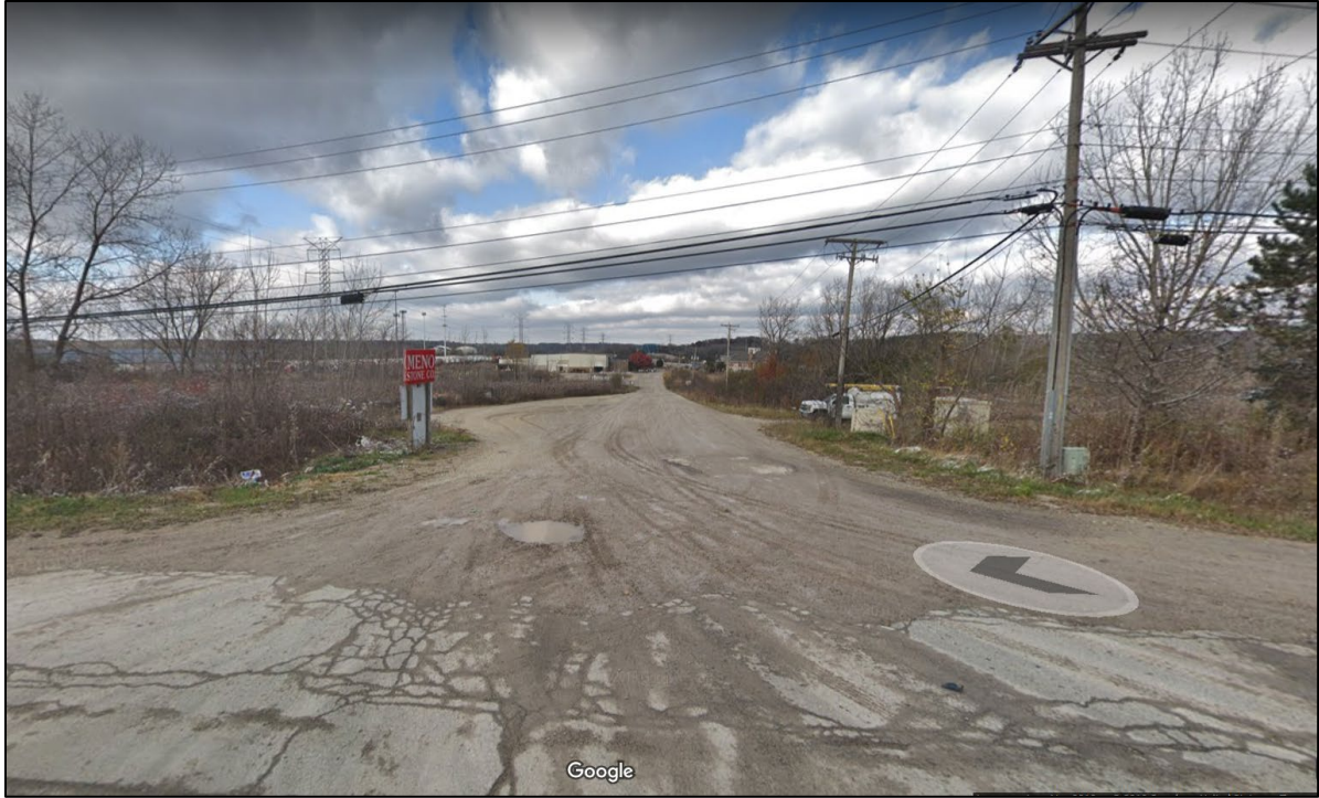
Figure 6: Looking north from Main Street at proposed M-1, Light Industrial segment of subject property.
