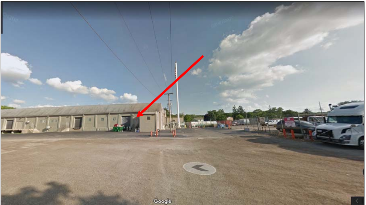
Figure 4: View of Unit 12 and its dock door
