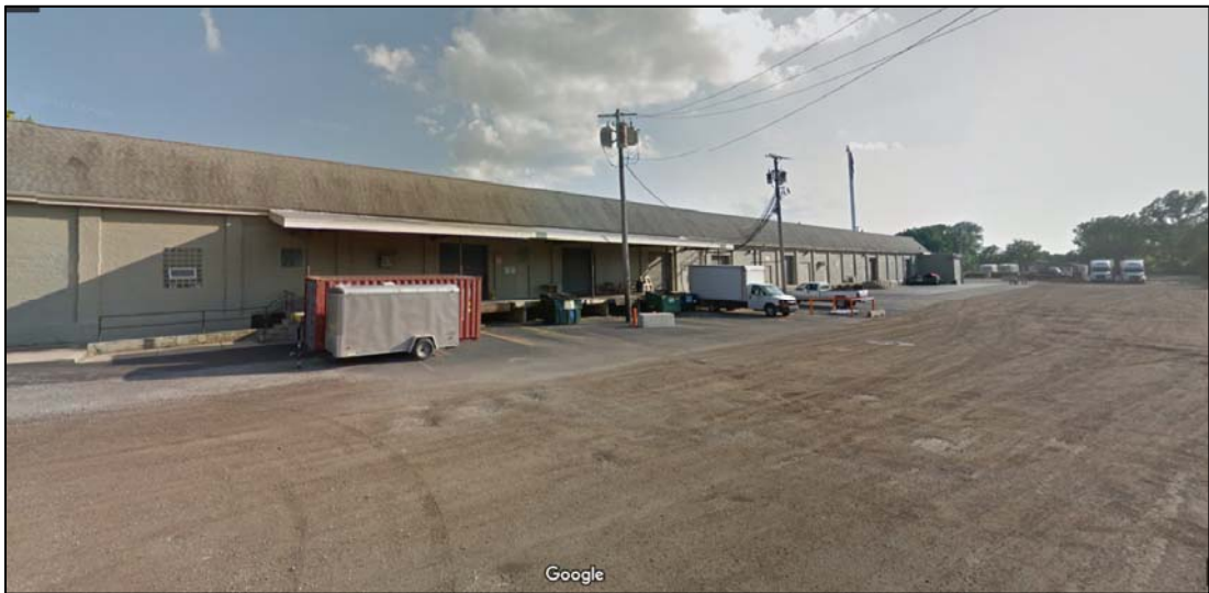
Figure 2: Rear of building looking southwest at loading dock area
