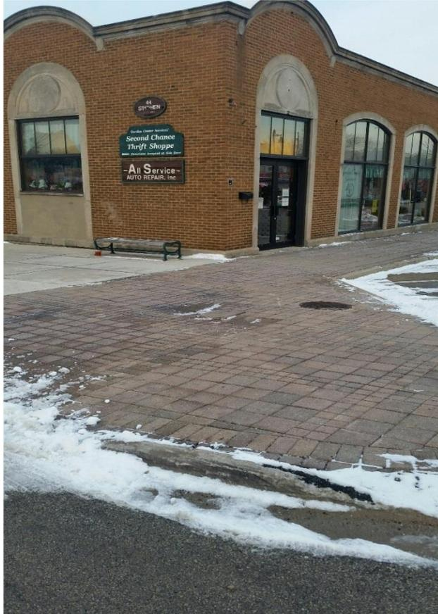
**Description:** Replace brick pavers on Stephen St. to match the new pavers on Main St. and Canal St./ Replace 21,000 SF of brick pavers on Stephen St., from Illinois St. to River St.
