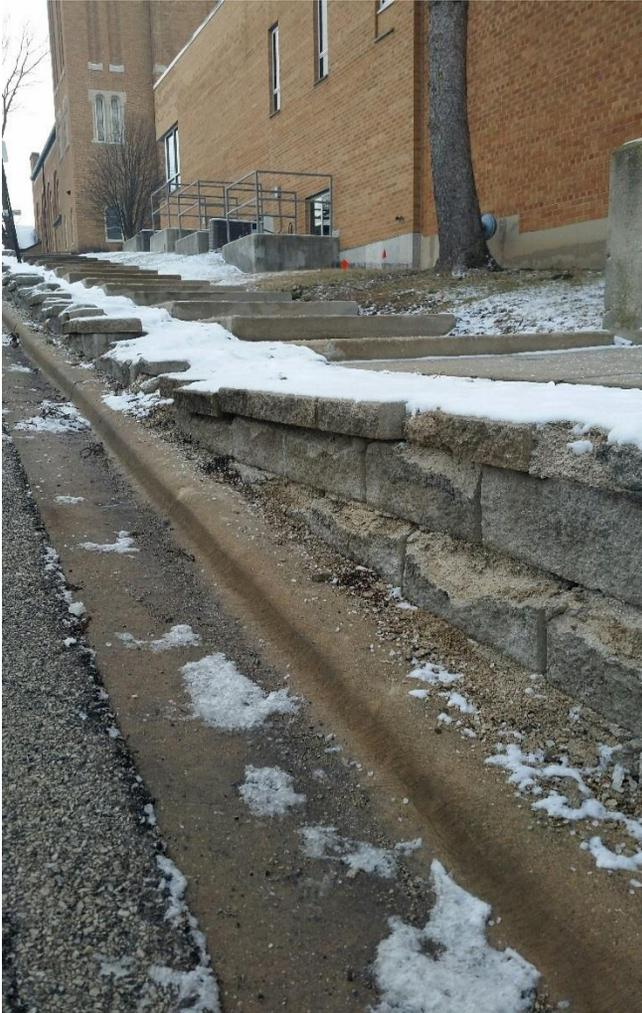
**Description:** Replacement of road salt deteriorated retaining wall along Czacki St., near Sobieski Street.
