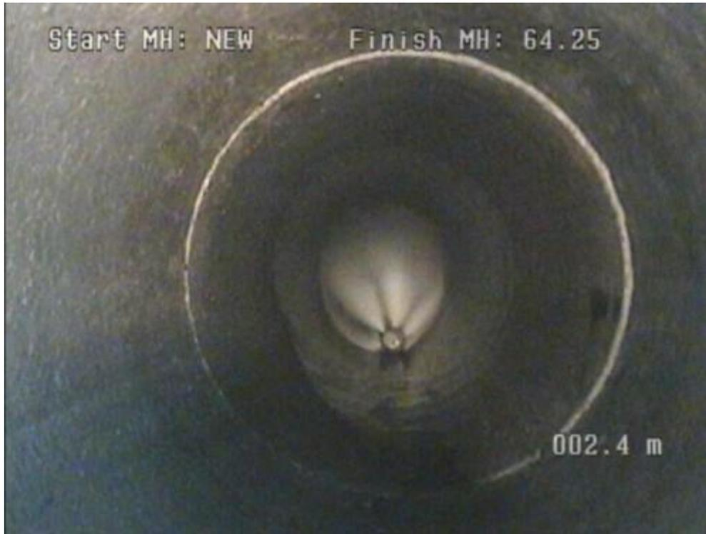
**Description:** Cleaning and televising of existing sanitary sewers and combined sewers, in order to maintain sewers in good, clean condition and to comply with recommended long term control plan.
