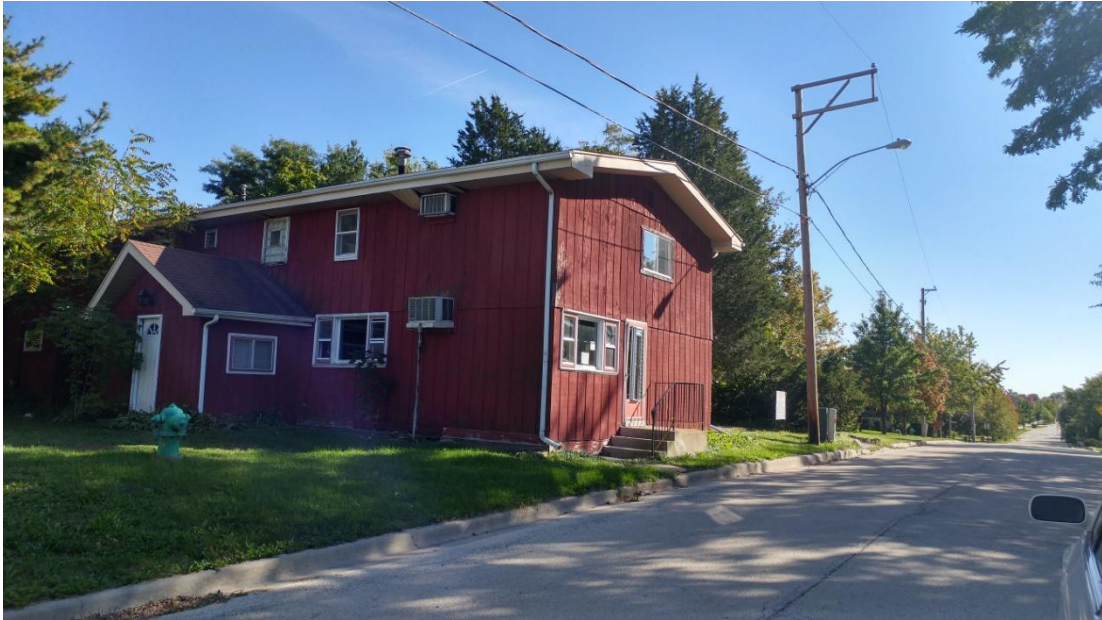
Photo 2 The view of the existing three-unit building looking south.
