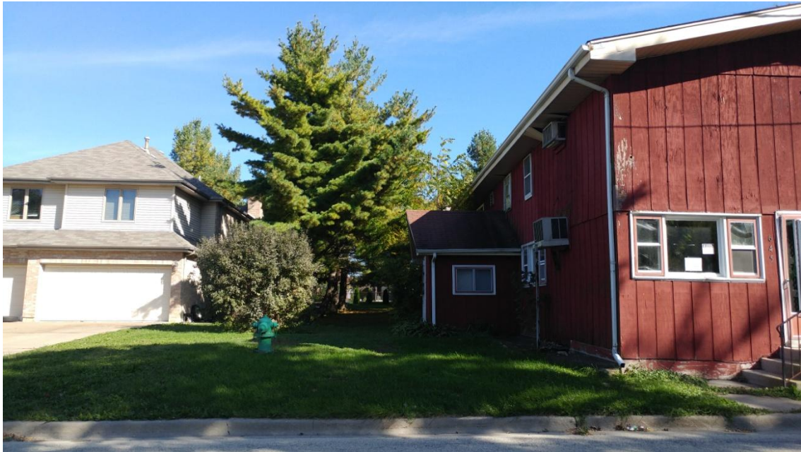
Photo 4 The neighboring homes are setback roughly 40 ft back from the street curb, which is significantly further setback than the three-unit building.
