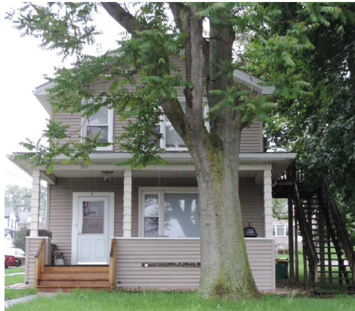
512 ILLINOIS ST - EXISTING
