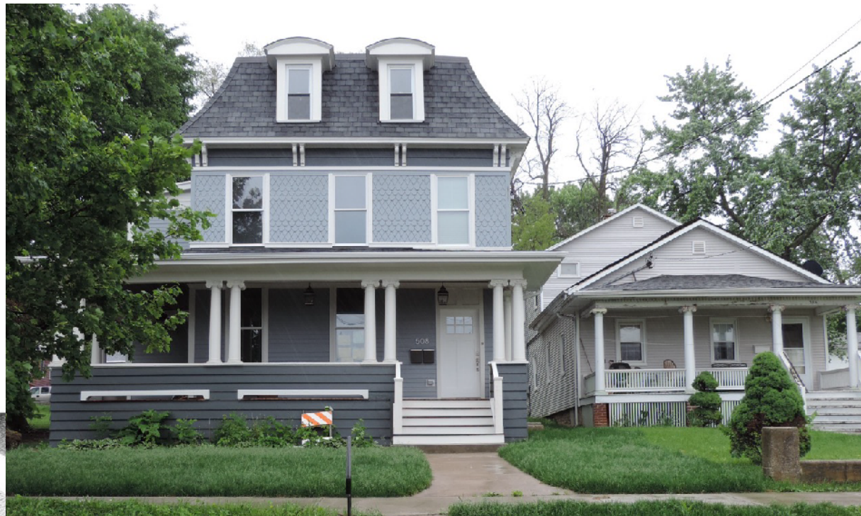
508 ILLINOIS ST - EXISTING
