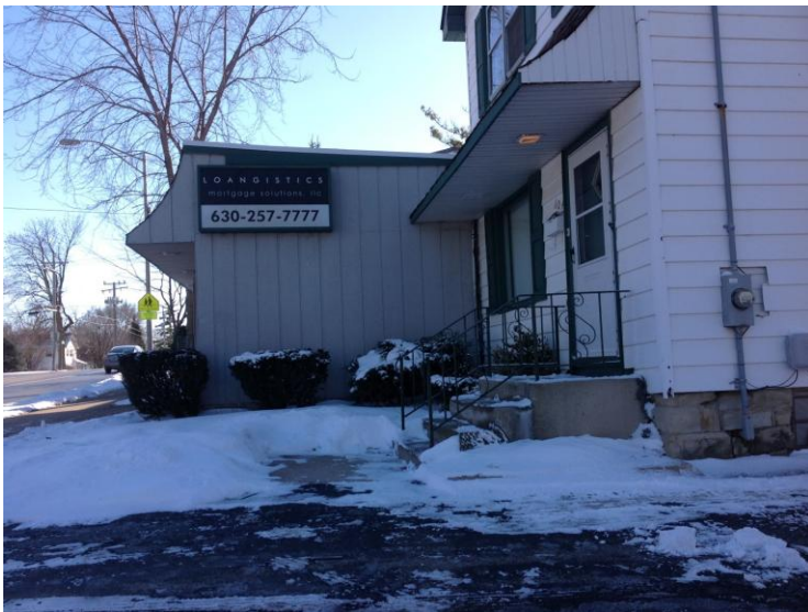
Nonconforming sign on the north facing elevation of the commercial structure.
