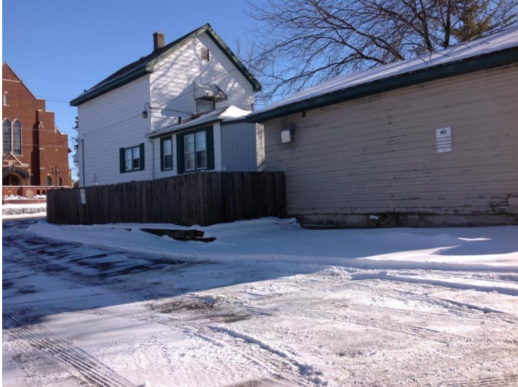
Residential structure and garage facing south east from the rear of the parking lot and alley.
