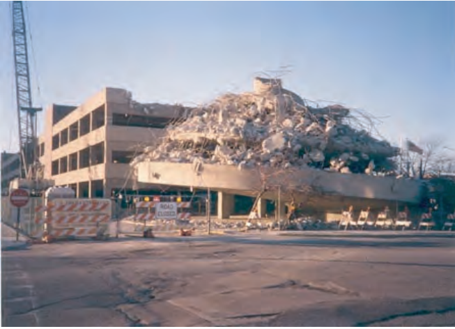
Figure 5. Deck demolition, Des Plaines, Illinois.
