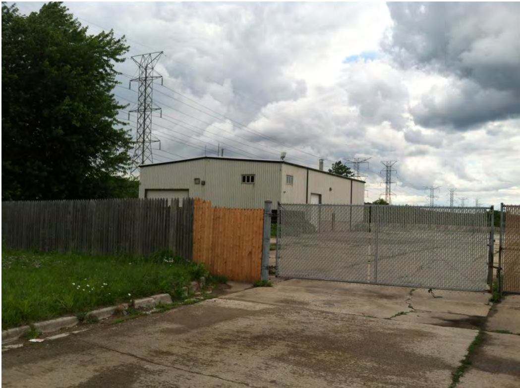
Facing East, at the subject property
