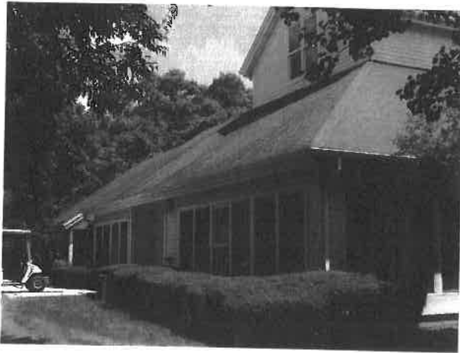
View looking southeast along north elevation of typical residential building (Building #1)
