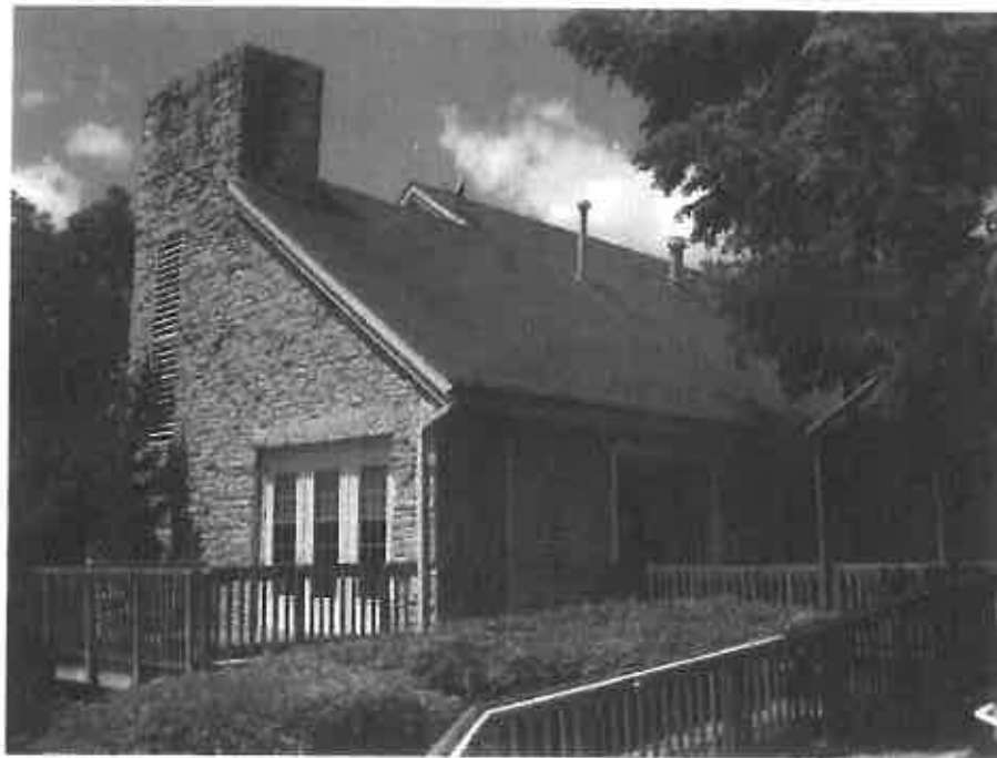
View looking northwest along south and east elevations of administration/office building (Building #6)
