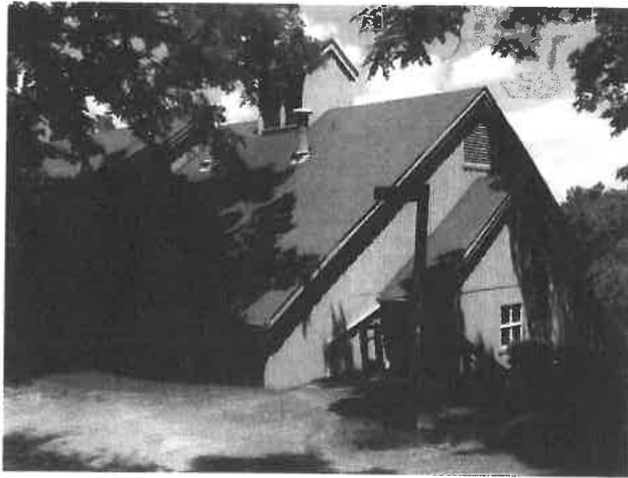
View looking northeast along south and west elevations of cafeteria building (Building #7)
