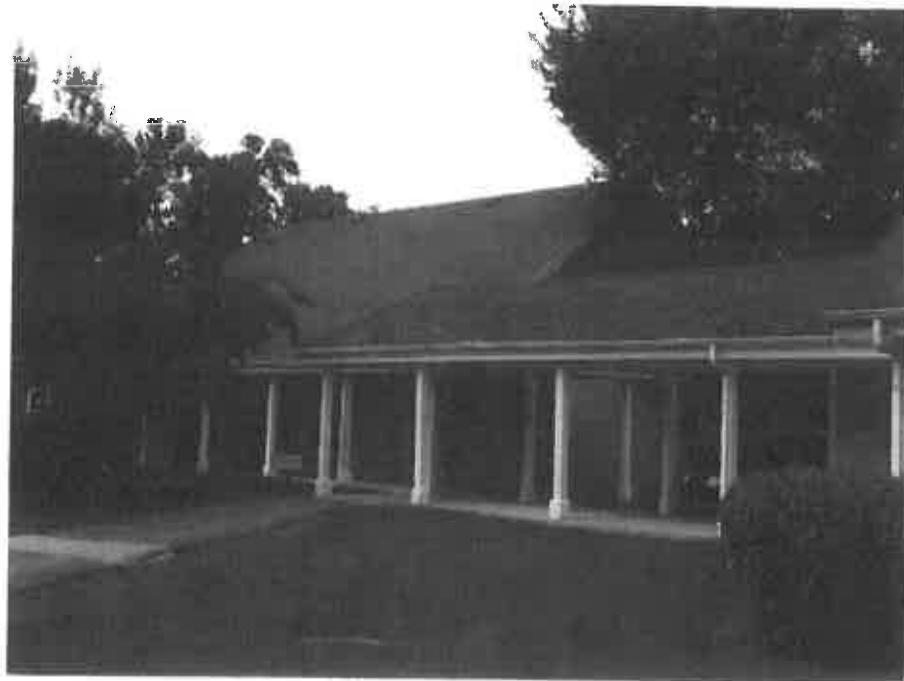
View looking west along south and east elevations of school facility (Building #4) showing connecting walkway to adjoining residential building
