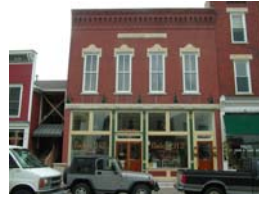
312 Canal Two-Part Commercial Block 1886 PS Hennebry, J. Hall Building IHSS-P; HABS
