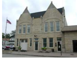
418 Main City Hall 1893 S Lemont Village Hall LMK; HABS
