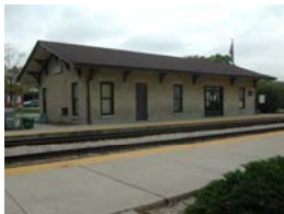
101 Main Railroad Station 1858 S Lemont Station IHSS-P; IHLS; LMK
