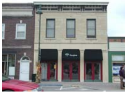
117 Stephen Two-Part Commercial Block c. 1865-67 S HABS
