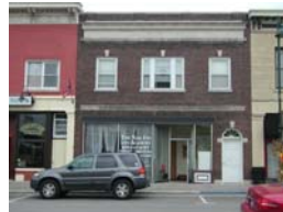
115 Stephen Two-Part Commercial Block c. 1924 S HABS
