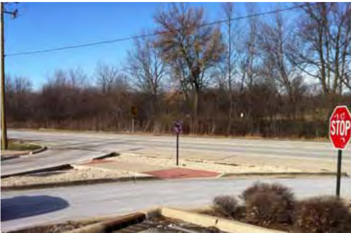
This stop sign and pedestrian island make it safer for pedestrians to cross the driveway at 3 Corners Shopping center. Adding a crosswalk would encourage drivers to check for pedestrians before exiting a shopping center.
