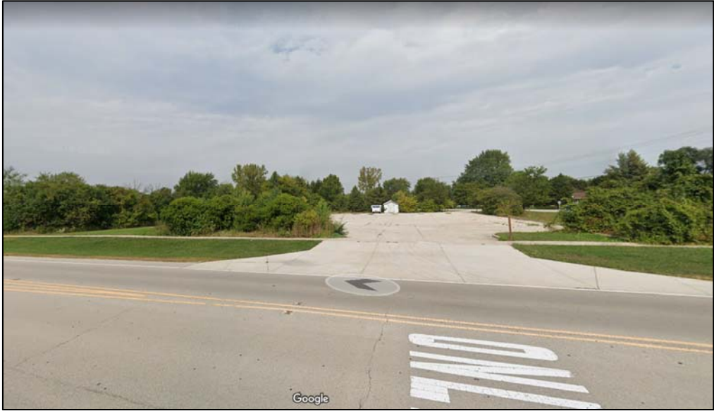
Figure 4: Streetview from September 2018 from McCarthy Road.
